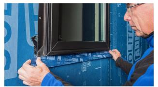
**18.1 Alternative: Sealing to flanged windows (USA)** Insert the window, fasten it and the seal with TESCON VANA on SOLITEX ADHERO all around the window in a waterproof manner. Rub the tape firmly using the pro clima PRESSFIX application tool to secure the adhesive bond.
