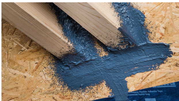
9. The finished joint at a double collar tie penetration
