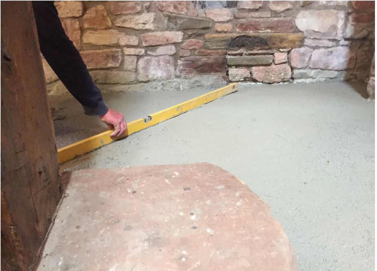
Above, A solid robust floor is achieved with Diathonite Cork Lime Screed Below, Diasen Thermactive Insulation applied to the walls
