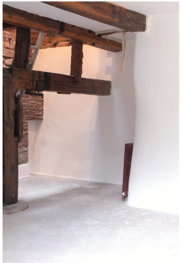
Above, A solid robust floor is achieved with Diathonite Cork Lime Screed Below, Diasen Thermactive Insulation applied to the walls
