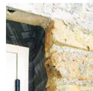
Thermal bridge free window installation with PHONOTHERM 200
