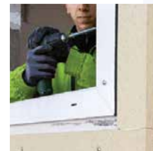
Thermal bridge free window installation with PHONOTHERM 200
