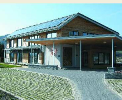
Courtesy JPW Construction
