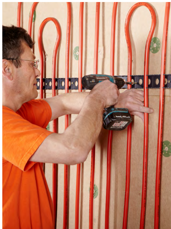
Fastening a hydronic heat element
