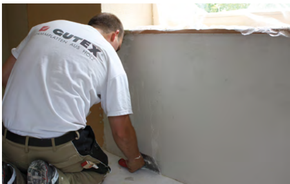
Application of final render
