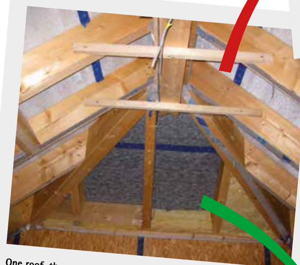
One roof, the same conditions, different results: pore-free SOLITEX PLUS membrane on the hip roof, microporous membrane on the main roof surfaces to the left and right.
