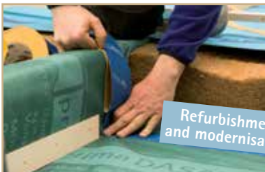
Interior air sealing
