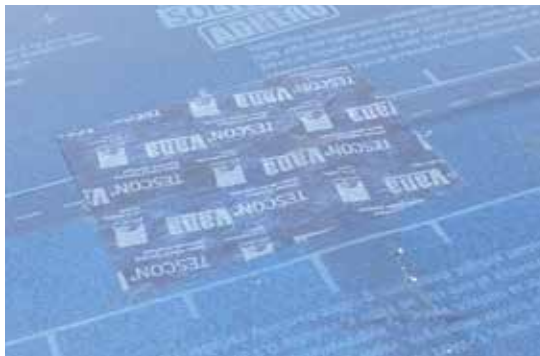
For sealing damaged areas on membranes.
