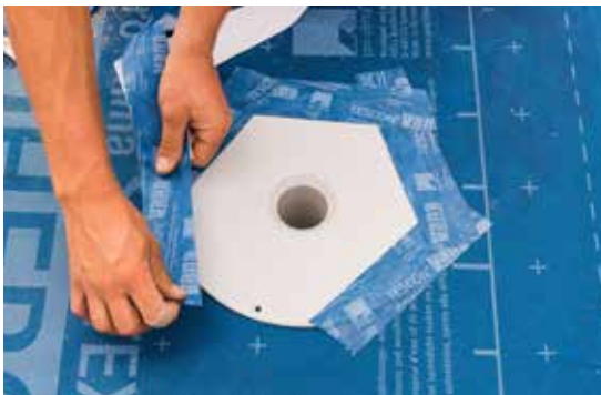
For creating seals between surface-drainage gullies and SOLITEX ADHERO.
