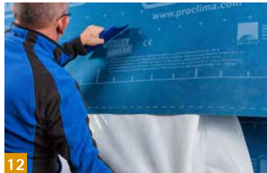
PRESSFIX XL Can be used to press SOLITEX ADHERO 1000/3000 into place easily and quickly
