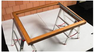
**1. Masonry or timber structure** CONTEGA SOLIDO EXO-D is to be applied before the window is installed. The frame is laid out flat with the exterior side facing up.
