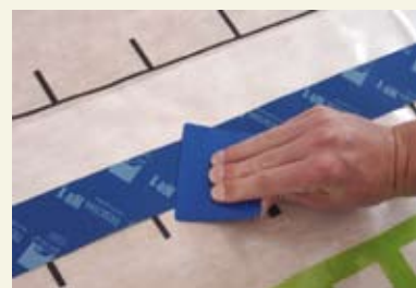
TESCON No.1 Multi-purpose adhesive tape for sealing membrane overlaps.
