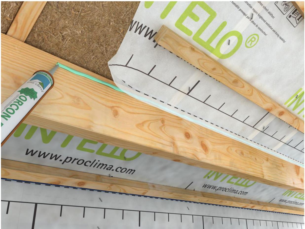
Figure 1: Bonding INTELLO to timber beam using ORCON F
